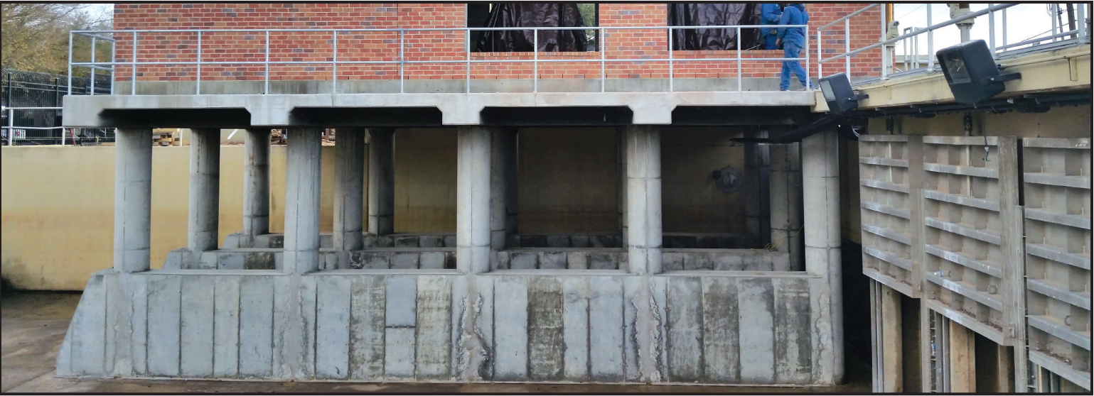
Pump Station F - Elevated Building Foundation
